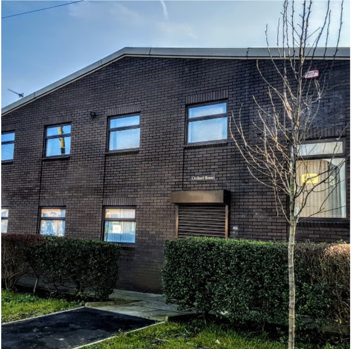
Orchard House, Hempshaw Lane, Stockport
